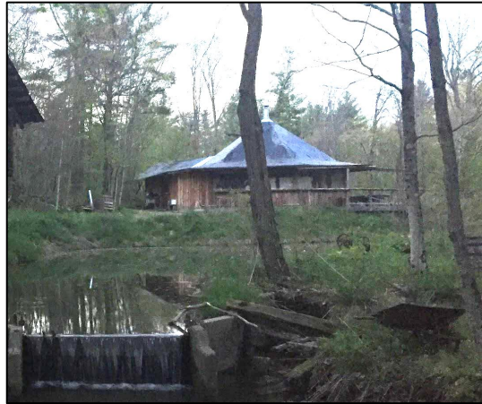
The Crown Jewel The final project the owner worked on. The "Purple People Heater" in the indoors, a wood fed stove to keep the place warm in the winter, is pictured on the next page. Photo Courtesy of Jack Castle
